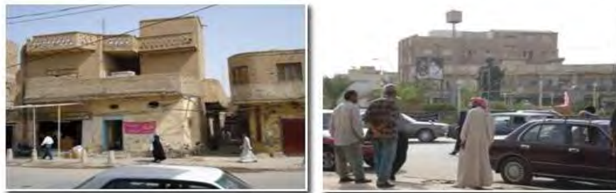
Picture (9) the absence of clearancy in the constructional style of Al Habbobi plaza (Source: Researcher - field study)
